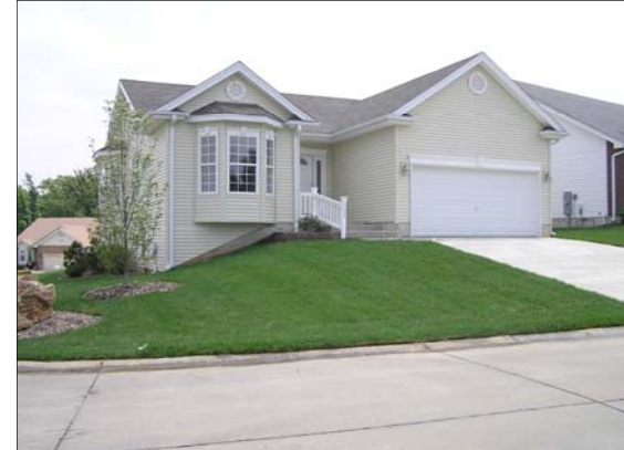
THE WASHINGTON Base Price $169,950 #208 FIDDLECREEK RIDGE RD Main Level 1,275 sq. ft. Lower Level 700 sq. ft.
